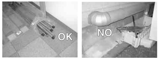
Store the pipes to be used indoors. (Warehouse at site or owner's warehouse) Storing them outdoors may cause dirt, waste, or water to infiltrate.
