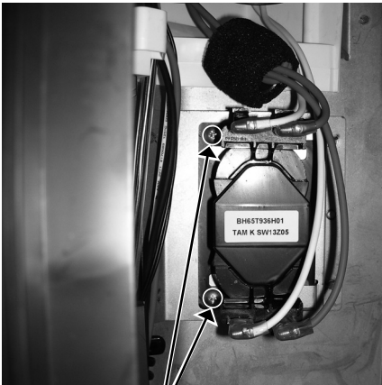
Screws of the reactor
