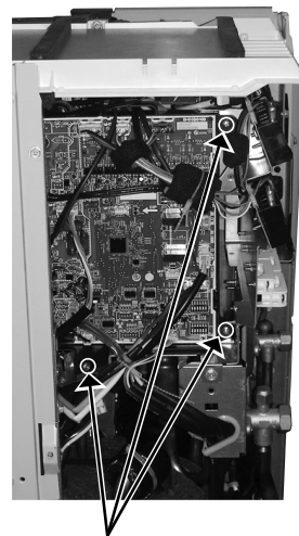
Screws of the outdoor control P.C. board holder
