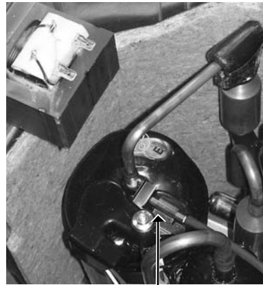
Discharge temperature thermistor
