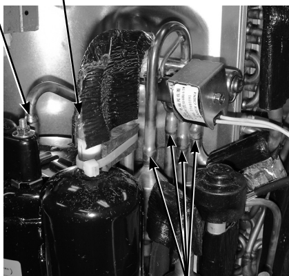
Brazed parts of 4-way valve
