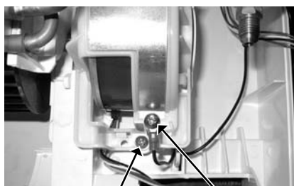
Screw of the motor band Screw of the earth wire
