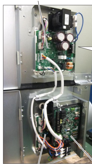
Power circuit board
