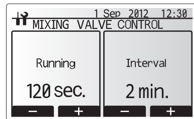
Mixing valve setting screen
