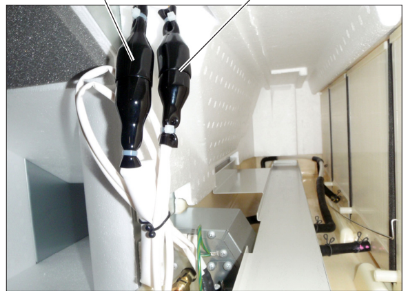
Connector for the solenoid valve Connector for the water sensor
